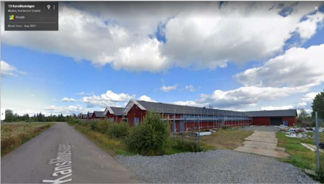
Figure 19 Screenshot of unfinished data center in Boden, Sweden, source: Google Maps
