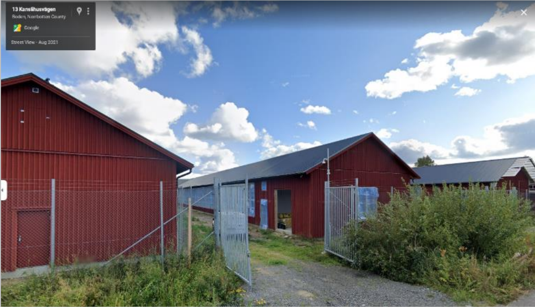
Figure 18 Screenshot of site in construction in Boden, Sweden, source: Google Maps
