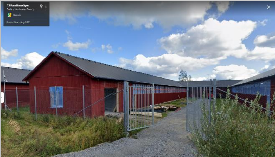
Figure 17 Screenshot of the facility in construction in Boden, Sweden, source: Google Maps
